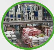
Cleaning & processing factory
